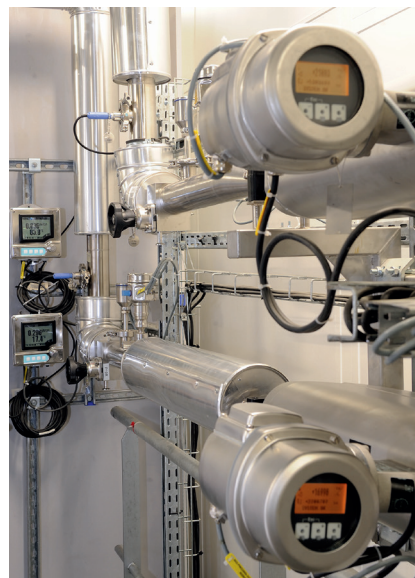
Flow measurement in WFI loop with Promass P.
