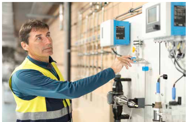
Analytical panels ensure high process quality and safety
