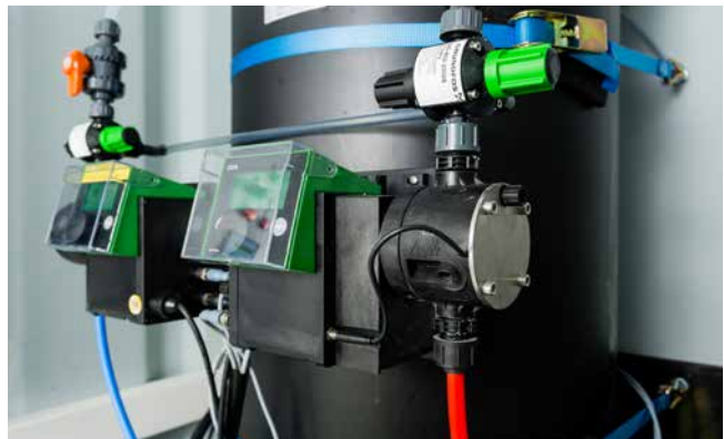
"Clorius2" chlorine dioxide generator for the safe and reliable disinfection of drinking water, cooling water and process water
