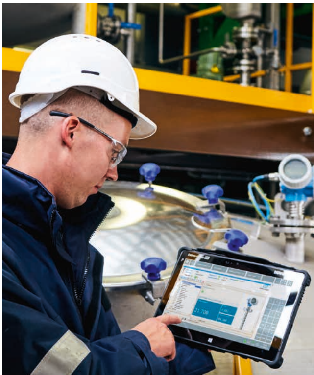
Contactless commissioning with a mobile device and the SmartBlue app
